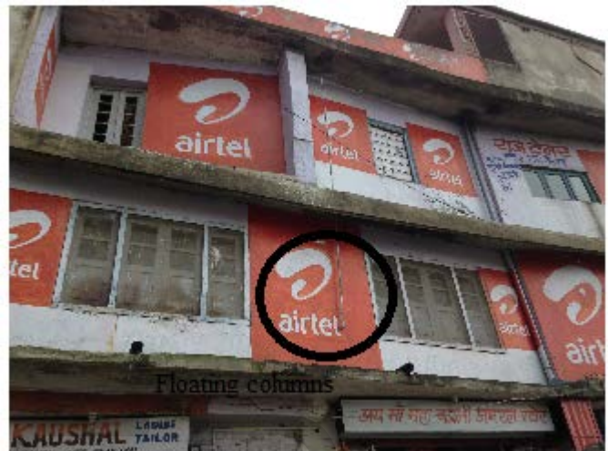
Fig . 6. Floating Columns
