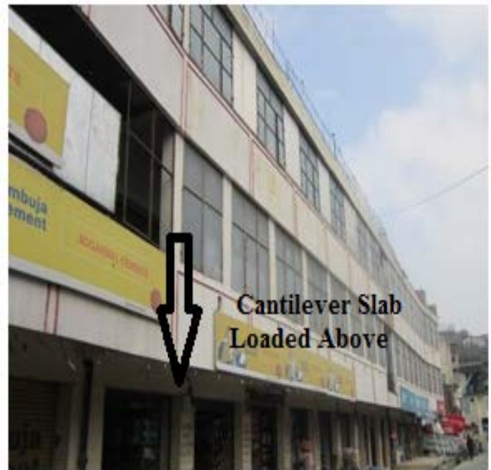
Fig.3 (a) Cantilever Slab Loaded Above
