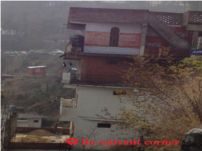
Fig. 7. Setbacks (Re-entrant corner)
